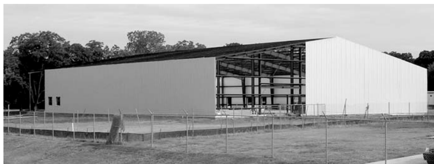
The Library Collection Depository, built during 2005, is a simple metal warehouse facility built on a concrete slab with temperature and humidity controls to protect the stored materials. The shelving will be 16’3” tall and will be arranged to accommodate the materials most efficiently. Eventually 300,000 volumes and more than 2000 boxes of archival material will be stored here.
